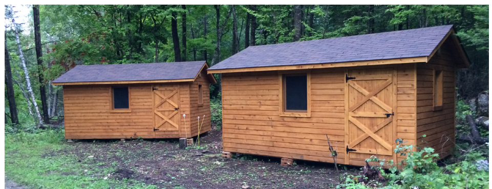
The staff cabins before the front decks were installed.
